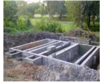
Establishment of constructed wetland system in progress.
