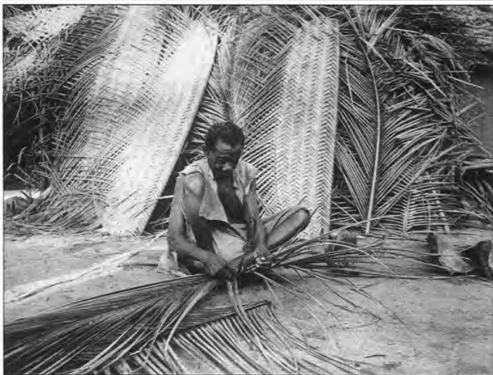
Plaiting of palm-leaves for roof covering. The art of building is founded on inherited knowledge. When building methods change, social and cultural patterns must also change.
