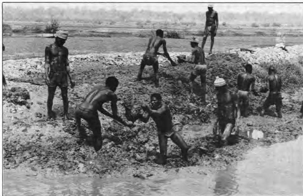
Manual construction of embankment
