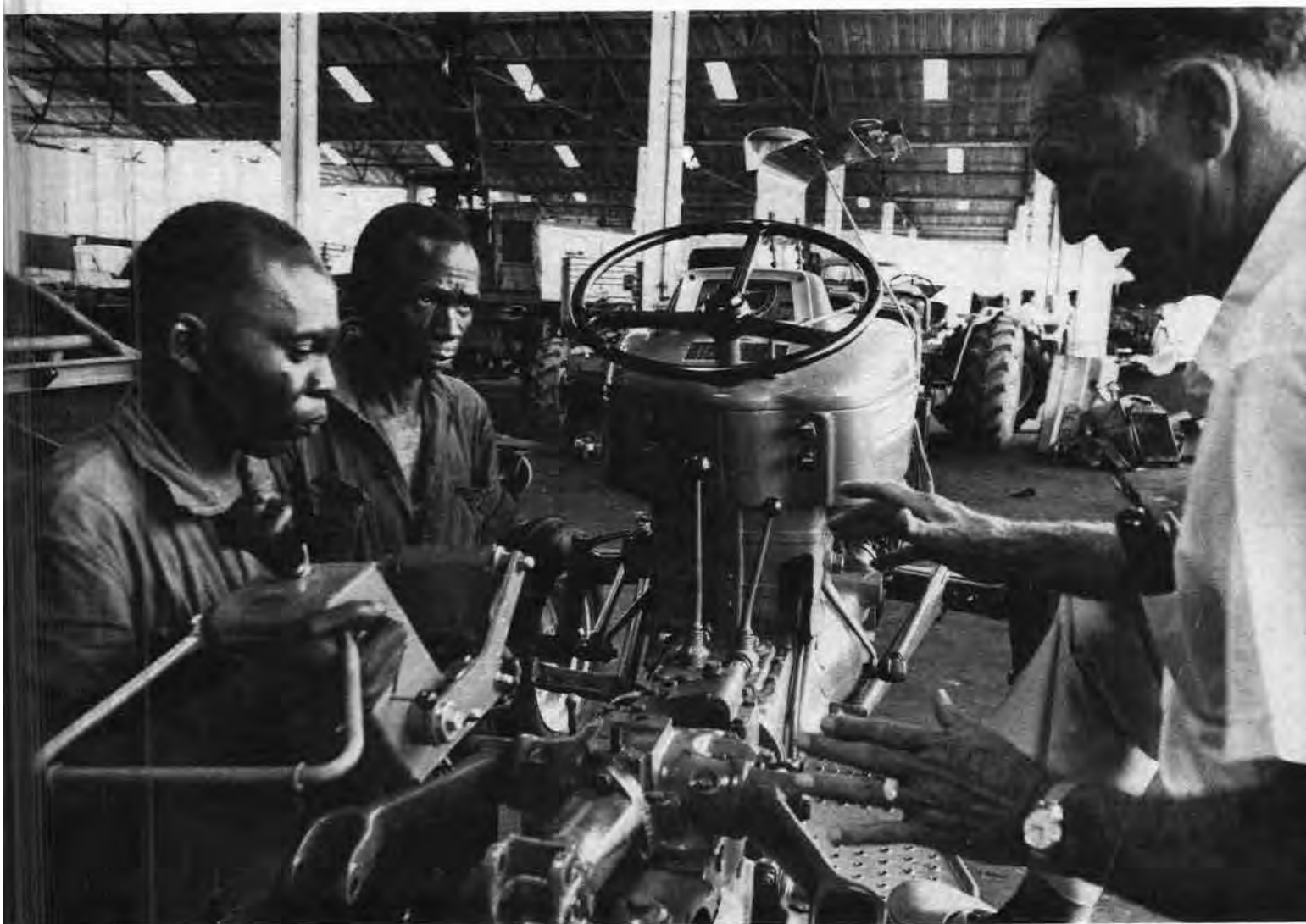
Trade testing on a tractor assembly, National Vocational Training Programme, Tanzania
