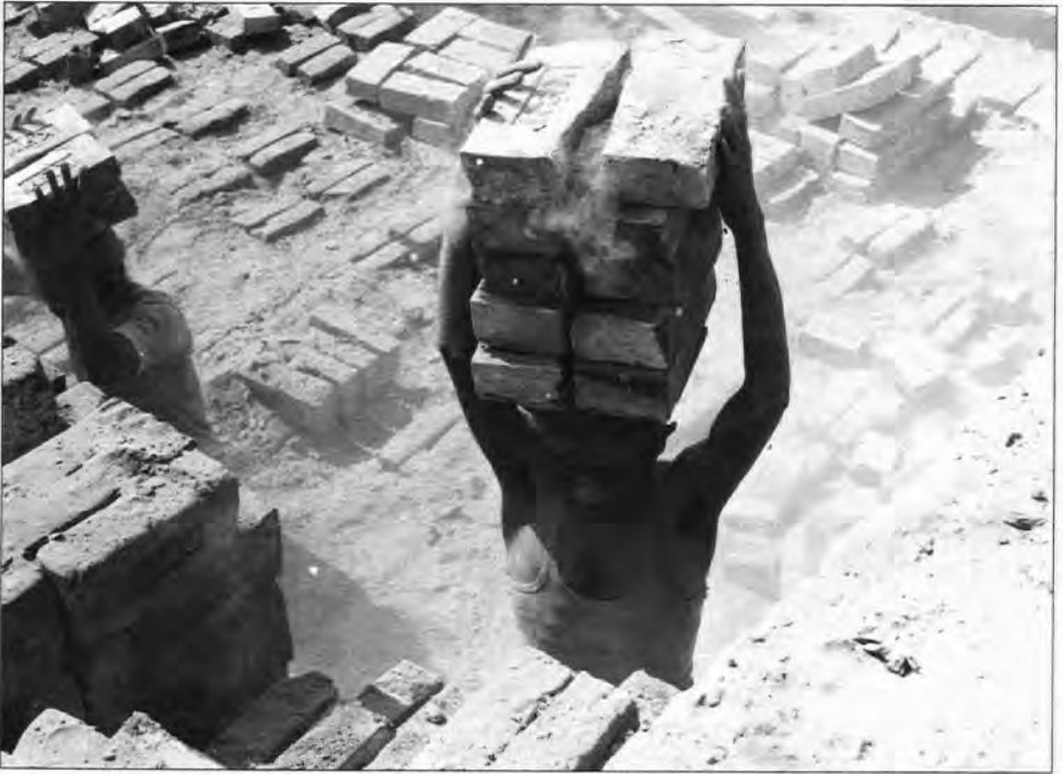
There is very little rock in Bangladesh. Instead bricks are used in road foundations. Here bricks are carried out from the brickworks. Photo: Brita Åsbrink, SIDA Photo Archives
