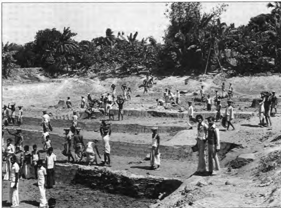
IRWP work-site. During the low season for farming the landless are given work in dam or road construction. Photo Eva Asplund, SIDA Photo Archives.
