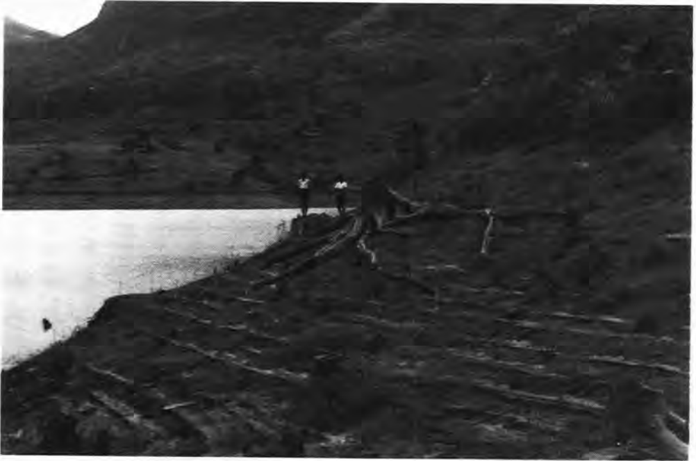
7. A rather steep section of a shore near Muslimgama. Abrasion has removed a layer of the topsoil exposing the root system of the felled trees. Coarse sand washed out by the waves is deposited in thin parallel stripes reflecting different levels of reservoir draw-down. January 15, 1988.
