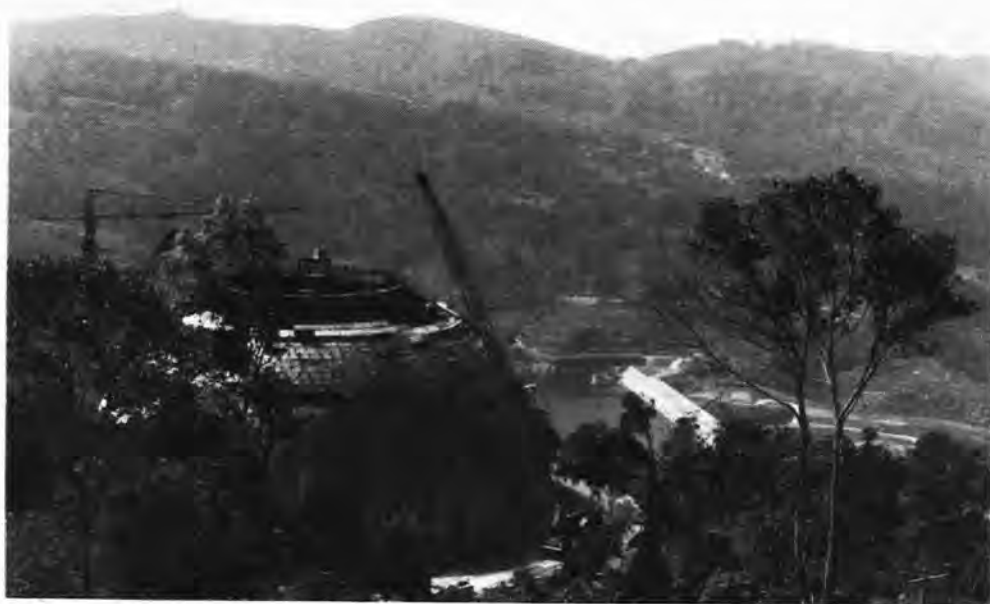
4. A very large dagoba under construction on the slope above the Kotmale dam. It has a diameter of 200 feet at ground level and the dome will have a height of 100 feet, on top of which a 173 feet, high "spear" will be placed. January 20, 1988.
