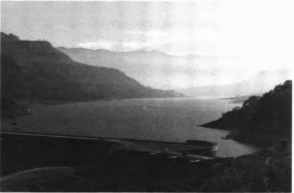
2. Kotmale reservoir at the damsite, January 22, 1988.
