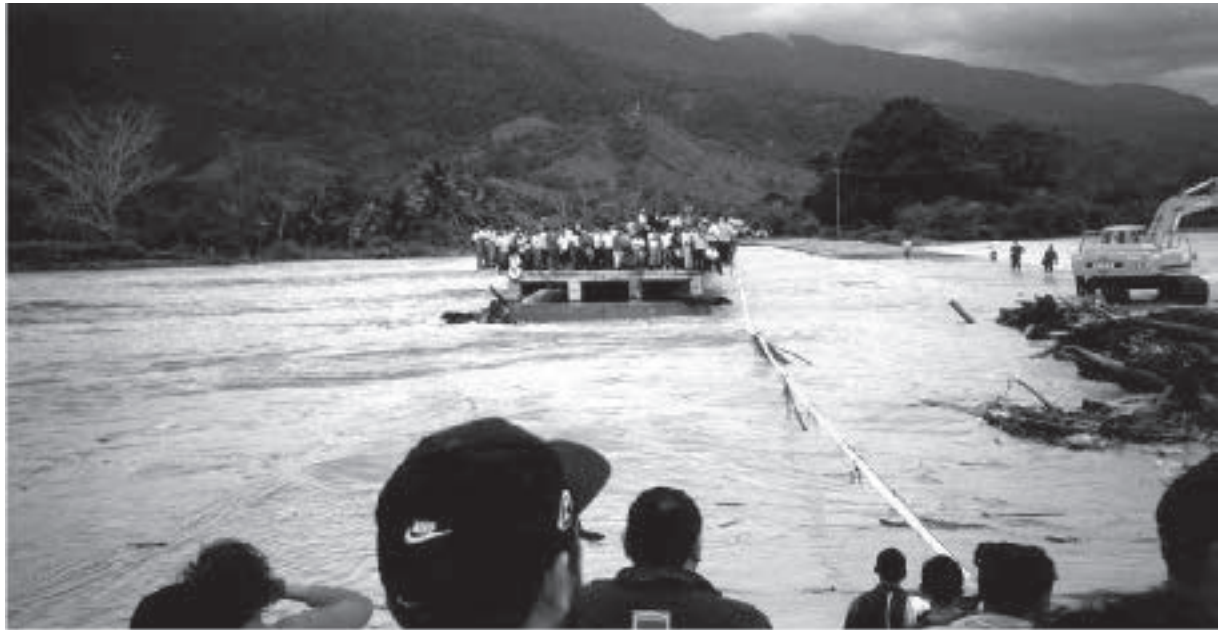
Phase 1: No crossing possible. Saba bridge. Source: SWECO
