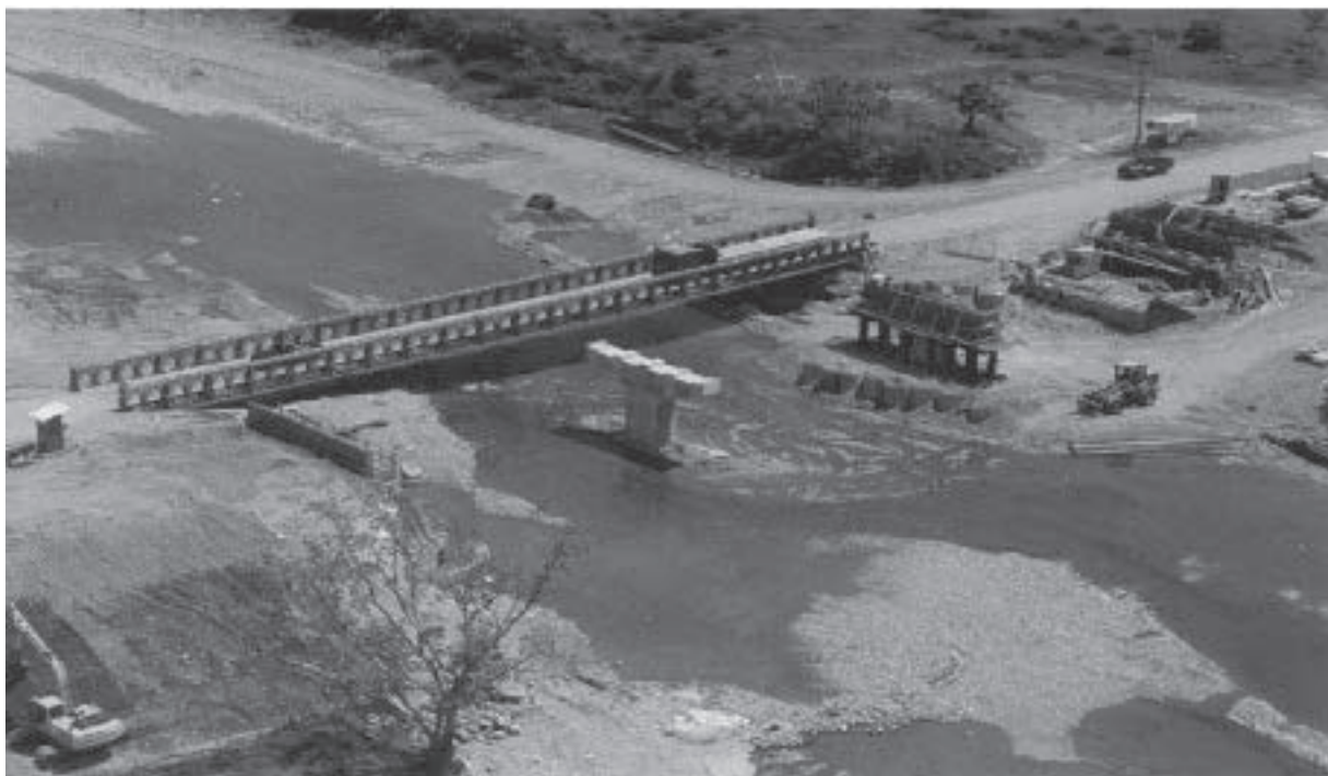
Phase 3: Bailey bridge at Bonito. Source: SWECO
