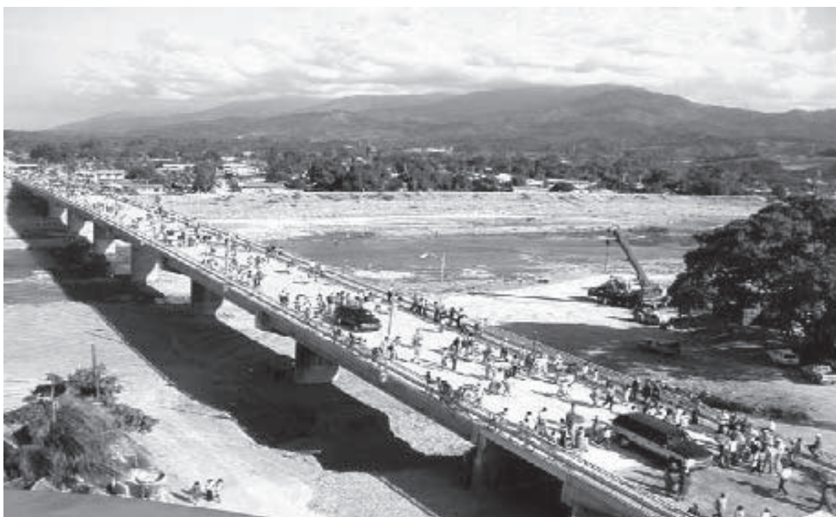
Phase 4: Reconstructed bridge Reino de Suecia at La Ceiba. Source: SWECO
