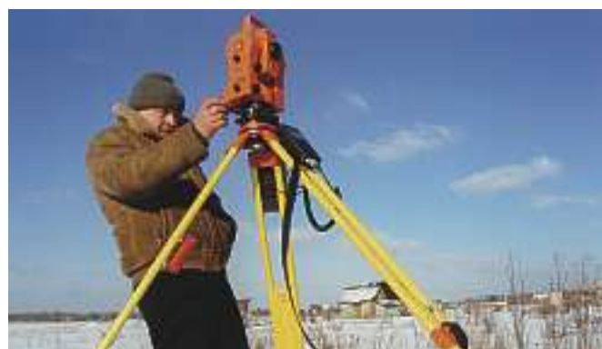
Land survey is an important part of the cooperation.
