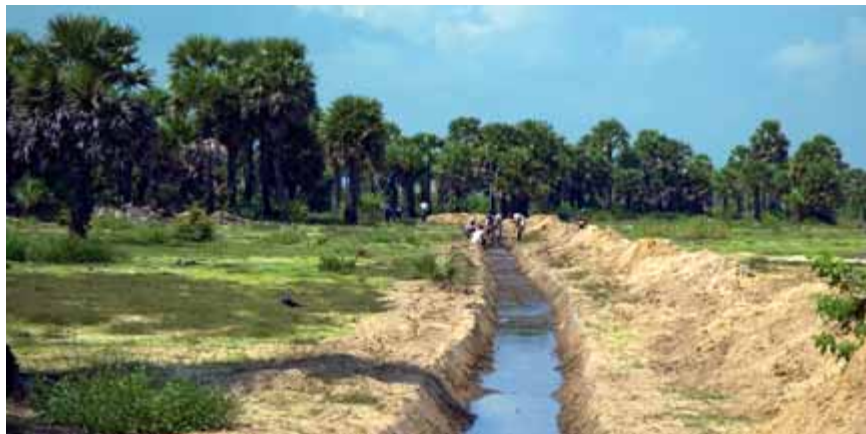
The ground has to be drained before construction can begin.
