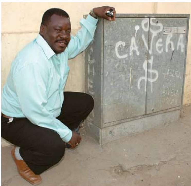
Domingos António, Edel, checks a distribution box made by Cerve
