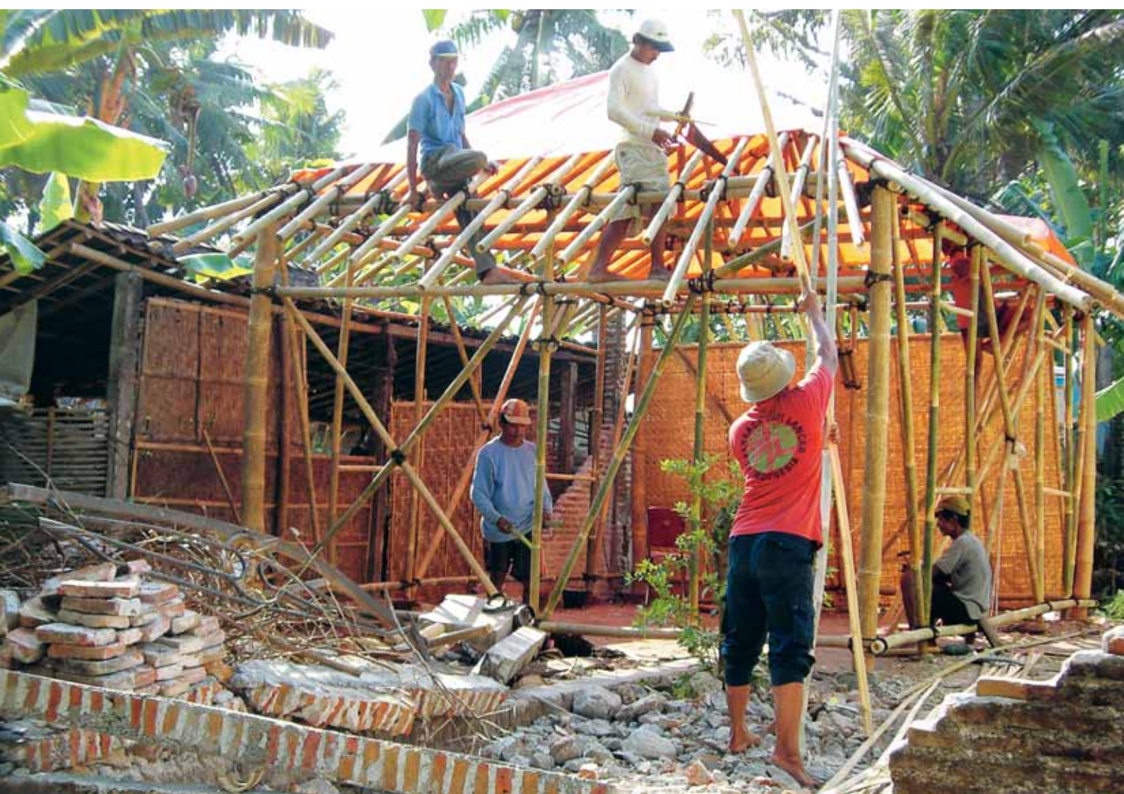
INDONESIA Sida provides support to IFRC for the construction of temporary houses after the earthquake on central Java in May 2006. The houses are built of bamboo using traditional building technology to enable them to resist future earthquakes.
