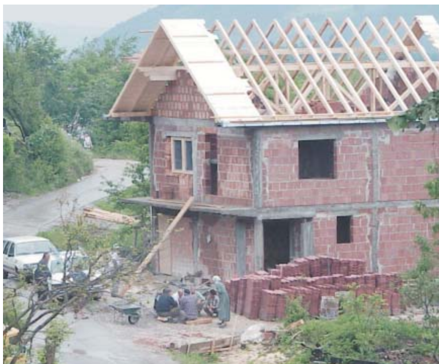
Returnees are assisted to rebuild their houses in the Sida-financed integrated area programs.
