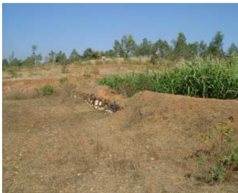
Photo 1: Some contour bunds tend to suffer from design or lay out deficiencies. This can be compensated to some extent by good maintenance.
