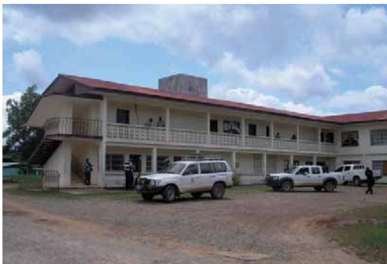
Rehabilitated administrative building, Sanniquelli city, Nimba county
