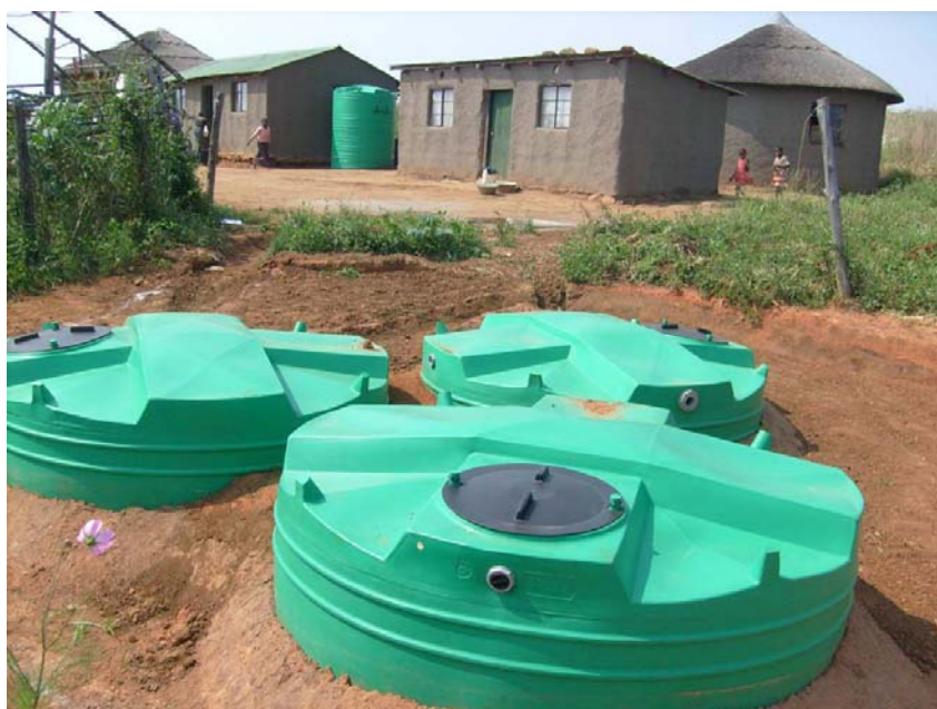
Figure 3.23: Plastic tanks (5,000 litres) installed in the Potshini catchment under a WRC funded project.
