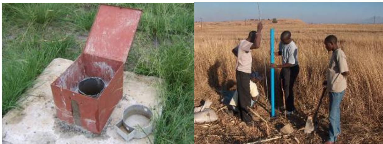
Figure 2.14: Installation of piezometers with Potshini High School pupils during their work experience week (left) and deep observation groundwater borehole (120 m deep, right).
