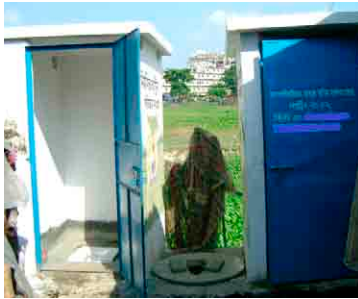
New public latrines have been installed in the north urban study area to replace these old ones but improper construction means they drain out into the nearby open space
