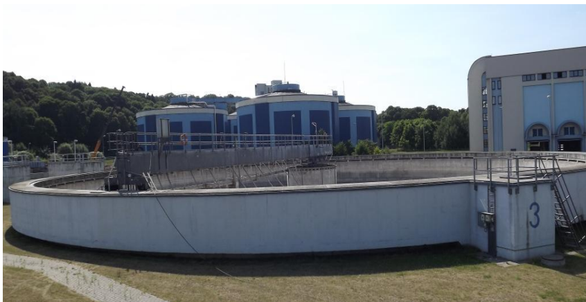
The picture above shows digesters, sludge dewatering building and one of four primary settling tanks from 1 st phase. The tanks were modified to the secondary clarifiers during 2 nd phase.
