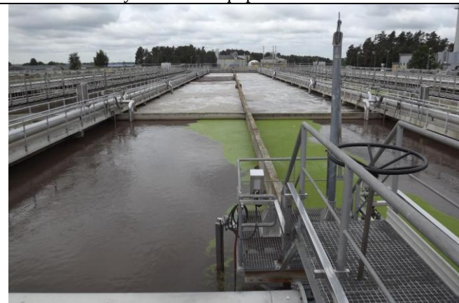
The picture above shows the activated sludge tank reconstructed in the 2 nd phase. In this case, green algae indicates that there are no toxic emissions from industry.
