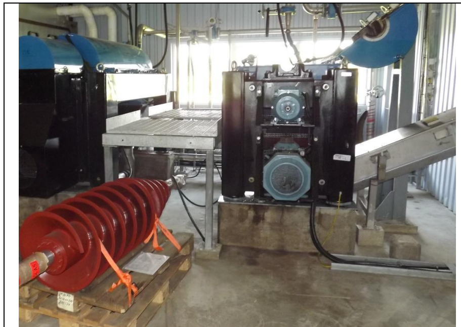
The picture above shows repair of the sludge centrifuge. The equipment supplied from Sweden. This is the first replacement of the rotor after installation.
