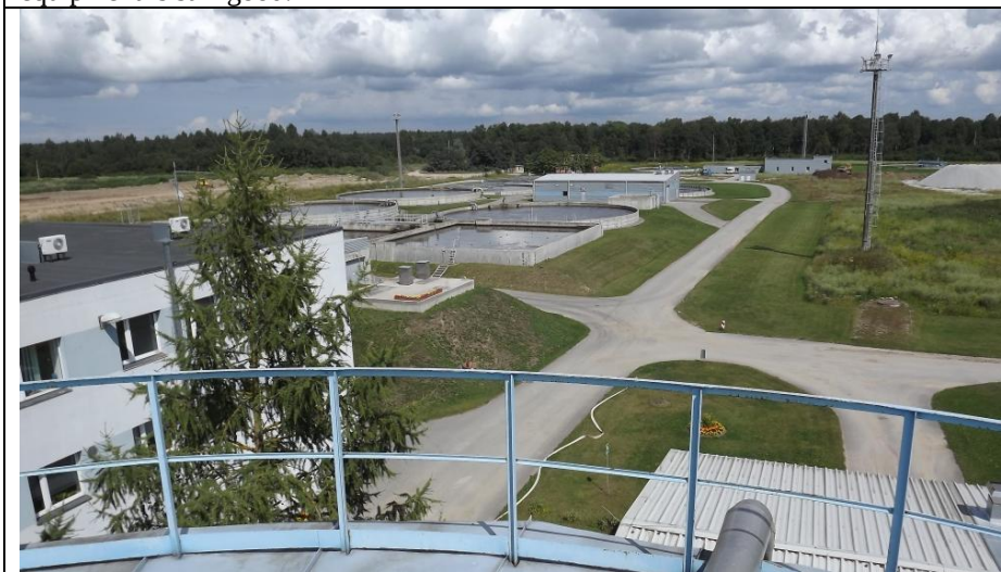
The picture above shows the plant layout from the top of digester. The plant includes separate municipal and industrial treatment lines.
