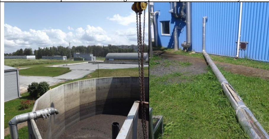
The pictures above show the sludge storage tank and bypass pipe done by water company. This is due to the reduced capacity of sludge digester (for reasons we don't know). Concrete tank is in good condition.
