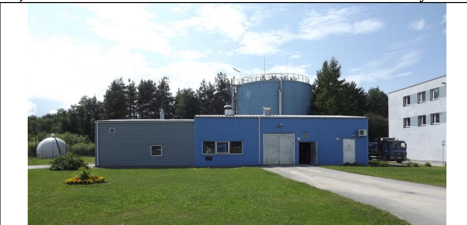
The picture above shows the sludge dewatering building, digester and gas holder. Dewatering intended for municipal and industrial sludge. This part of the plant was financed by Sida.
