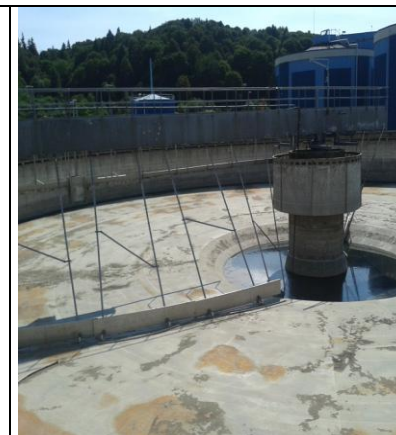
The pictures above shows yearly maintenance and cleaning of one of the secondary clarifier during summer season. The clarifiers were constructed at 1 st phase, concrete quality still very good. Later, at 2 nd phase the new sludge scrapers were installed in all of 4 tanks.
