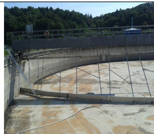
The pictures above shows yearly maintenance and cleaning of one of the secondary clarifier during summer season. The clarifiers were constructed at 1 st phase, concrete quality still very good. Later, at 2 nd phase the new sludge scrapers were installed in all of 4 tanks.
