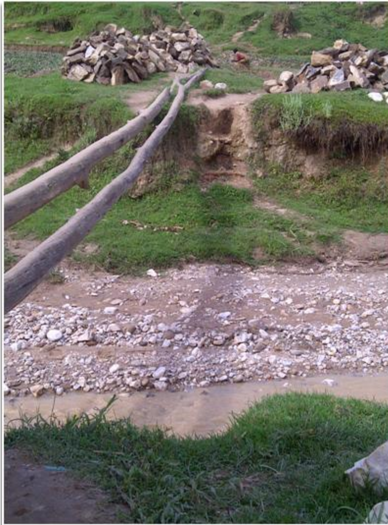
Stones that have been piled up in preparation for the construction of the long awaited for bridge
