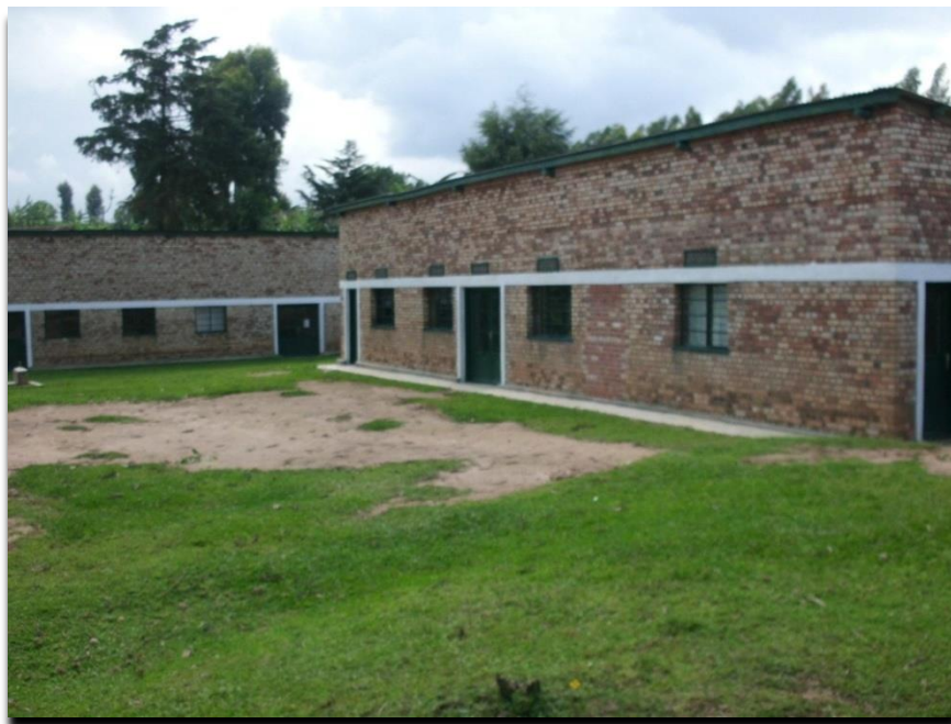
These buildings which were used for community literacy and numeracy programme have been renovated and currently house the Rwimbogo Health Post
