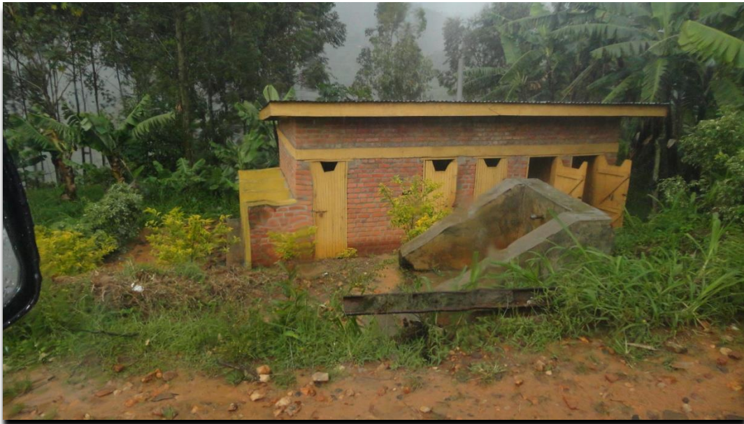
Maintaining these latrines clean is difficult because they are built outside the health centre's enclosure and hence used not only by patients but also by passers-by
