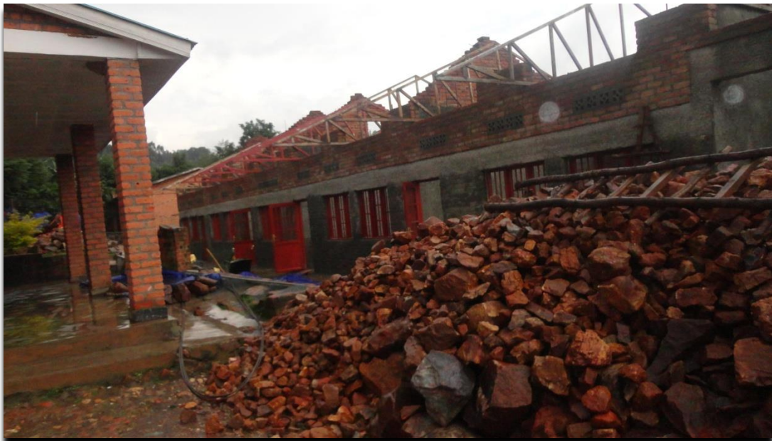
This bloc under renovation will house maternity among other services
