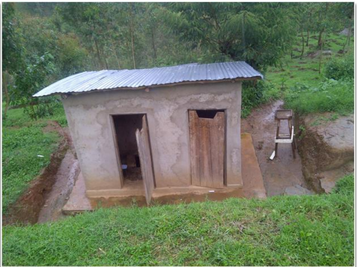
Two additional external toilets constructed in order to complement the ones that existed before at Nyange A Health Centre
