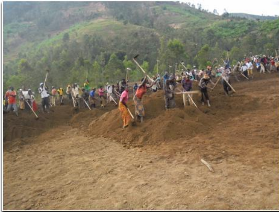
Citizens clearing the site where Muyongwe Health Centre will be constructed soon
