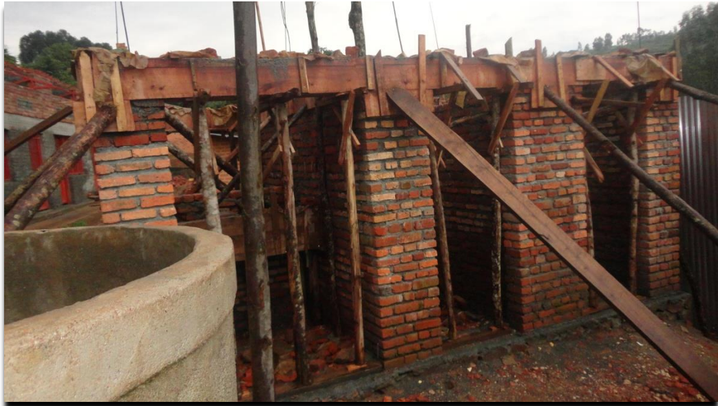
New latrines under construction within the health centre's compound
