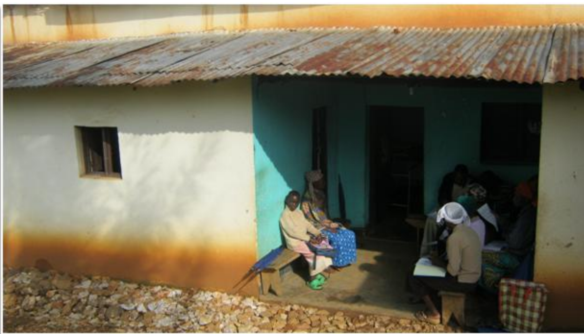
The above is the old building currently housing Ruhunga Health Post. People sitting in the veranda are community health animators compiling data for reporting
