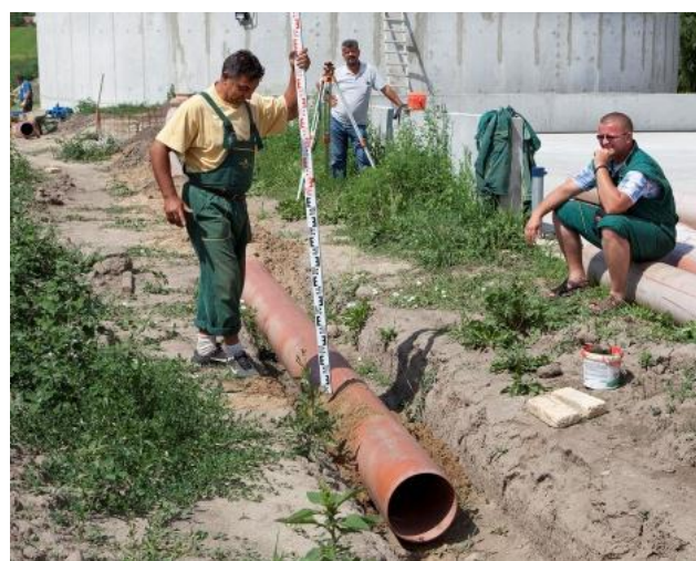
Improving wastewater treatment in Serbia through construction of a new plant. Photo: Victor Brott/Sida
