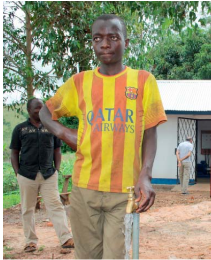
Mr Mwakajileke demonstrates the newly installed water pumping plant that supplies water to 6,000 villagers through 17 distribution points in a 6 km radius. Previously people would have to walk more than 1 km down to the river to collect their water.
