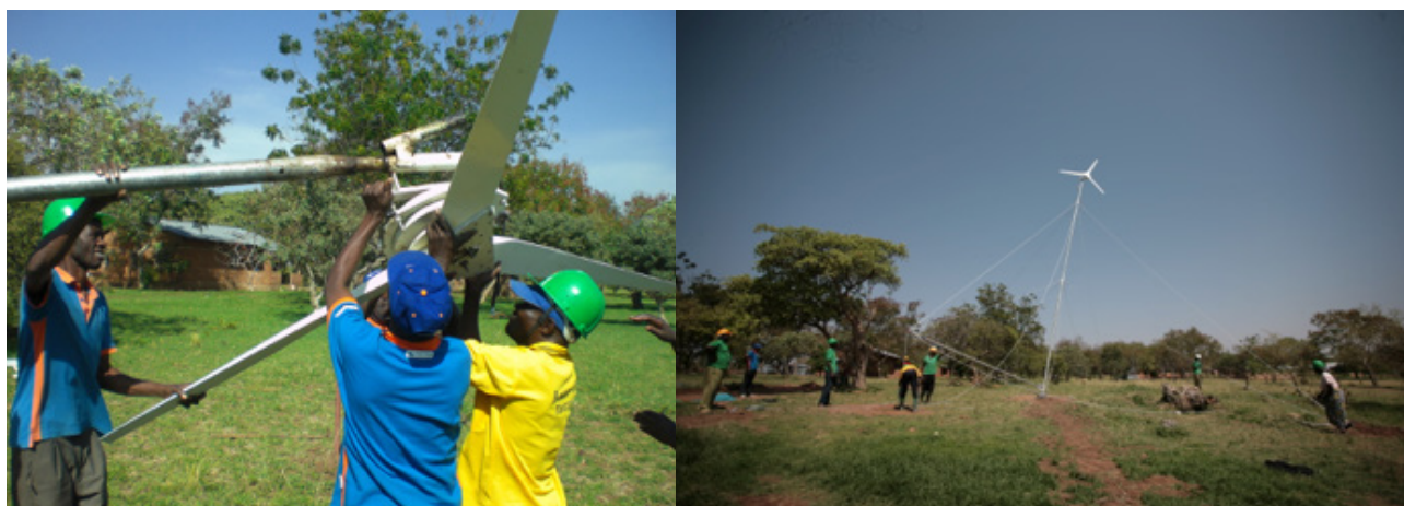
Figure 15: The Hugh Piggott wind turbine can be built locally and handled without machines.
