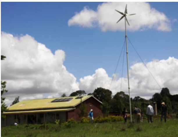
Figure 38: Quameyu Health Centre, 1 kW Wind power and 1 kW solar hybrid system with an integrated battery back-up.
