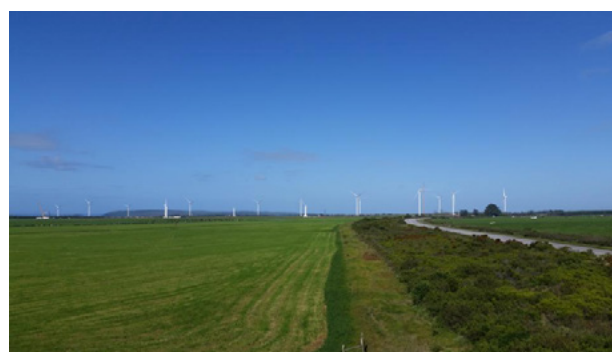
Figure 36: Cennergi Tsitsikamma Community wind farm project – 95 MW Wind farm built on community land in the Eastern Cape.
