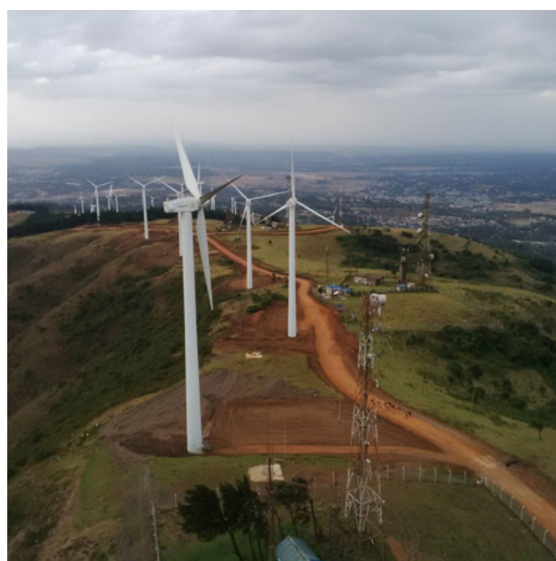
Figure 25: The Ngong II wind farm, with an installed capacity of 13.6 MW, is located 30 km west of Nairobi.
