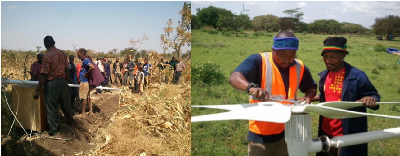
Figure 37: Villagers' participation in erection of the mast and assembly of the wind turbine assisted by the Change Agent.
