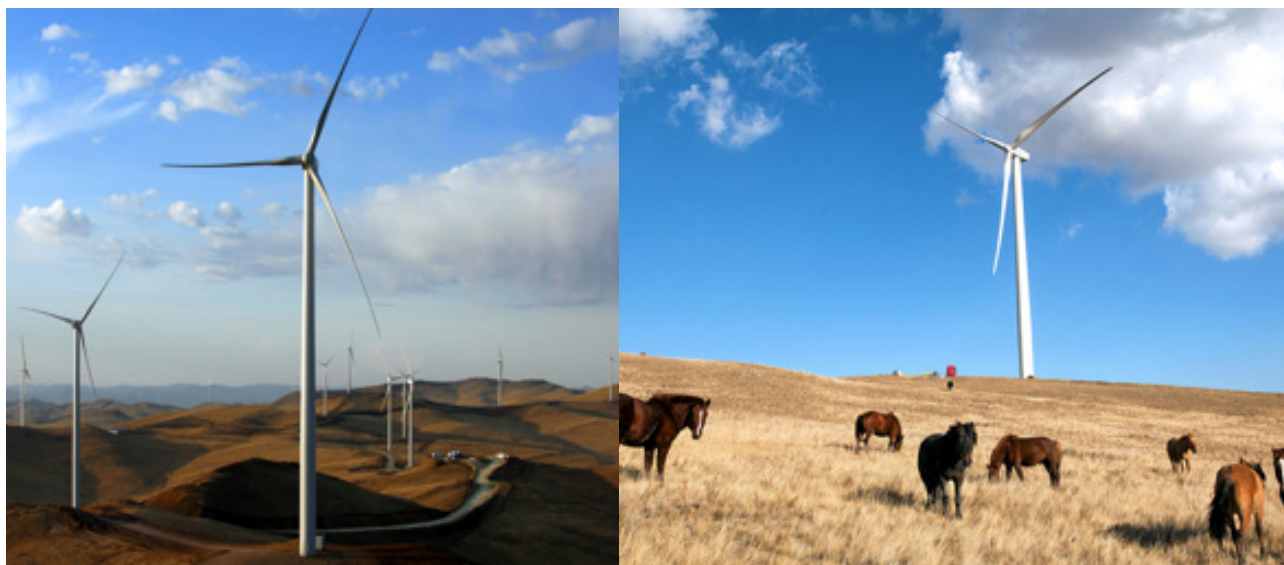
Figure 27: The first grid connected wind farm in Mongolia established by Public Private Partnership which has broken up the national monopoly. The project was undertaken in international cooperation with GE providing new technology. Due to the new feed-in-tariff policy the long term viability was secured.
